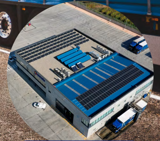
Solar panels in our HQ
